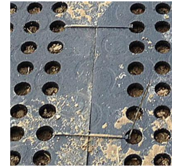
mats, attached to each other with cable zip ties
